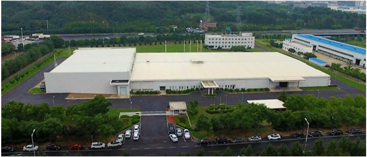
View of the plant to be transferred
